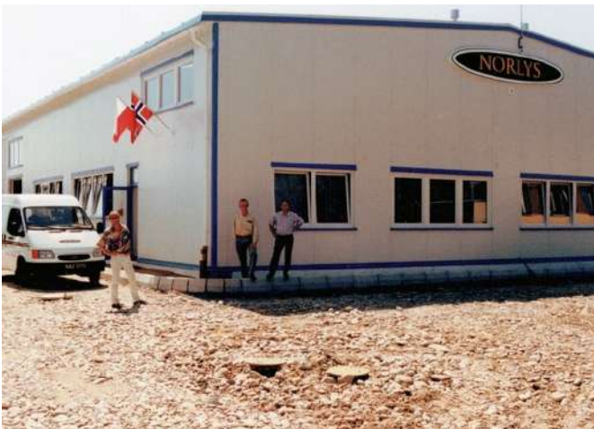
Brand new production hall (1998)
