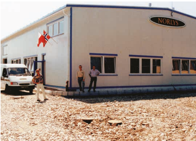
Brand new production hall (1998)
