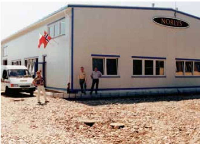
Brand new production hall (1998)
