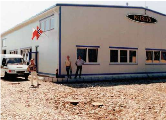
Brand new production hall (1998)
