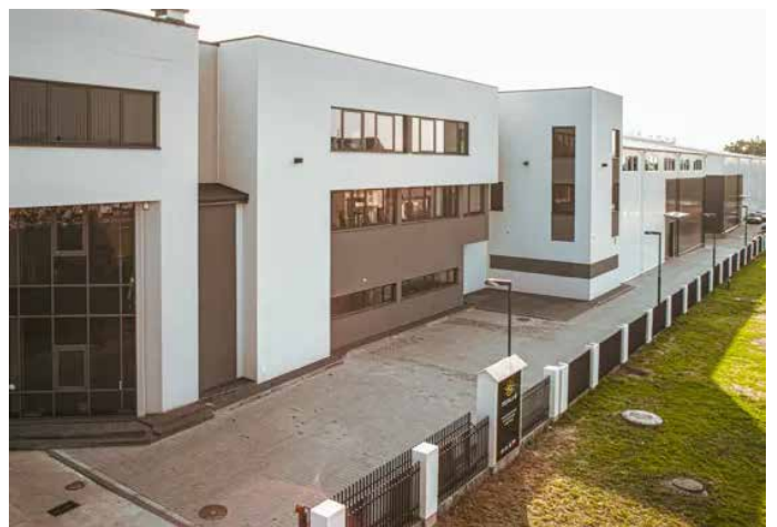
New warehouse and assembly (2015)
